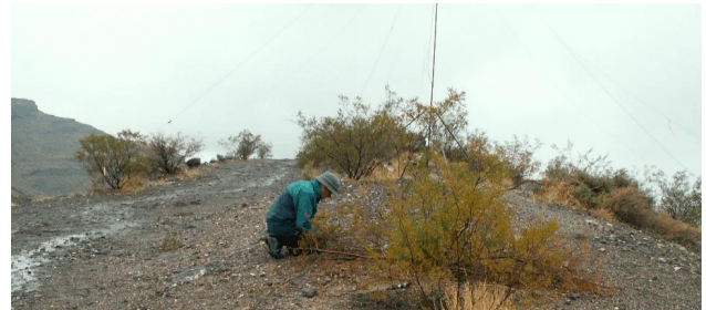
Norman replacing a water logged coax in the rain
